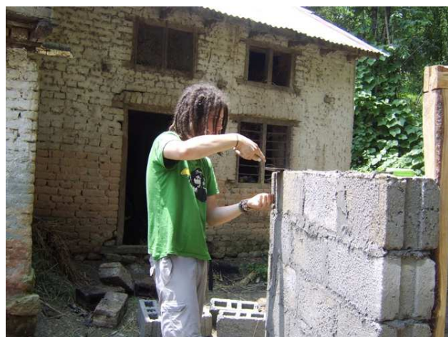
Volunteer constructing toilet
